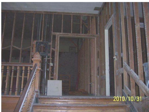
Entrance to Courtroom
